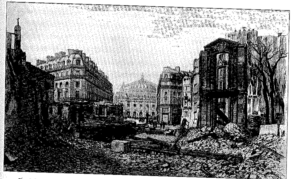
Fig. 3.2. Root shock in Paris. Compare with root shock in Pittsburgh, fig. 7.3, and root shock in New York after 9/11, fig. 8.5. Upper lithograph: Honoré Daumier. From the series "Locataires et Propriétaires": Scene from a neighborhood in process of demolition. REPRODUCED COURTESY OF THE PHOTOTHÈQUE DES MUSÉES DE LA VILLE DE PARIS. Lower lithograph: Demolition for the Avenue de l'Opéra. REPRODUCED FROM L'ILLUSTRATION , 1929.
