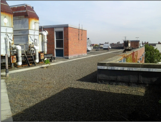
The eastern side of the Whitehead Hall roof.
