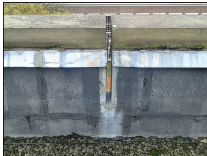
The pre-existing rain spout on the side of the Whitehead Hall roof. Our project involves lowering its base by five inches and then adding a second spout on the other side of the eastern roof wall.
