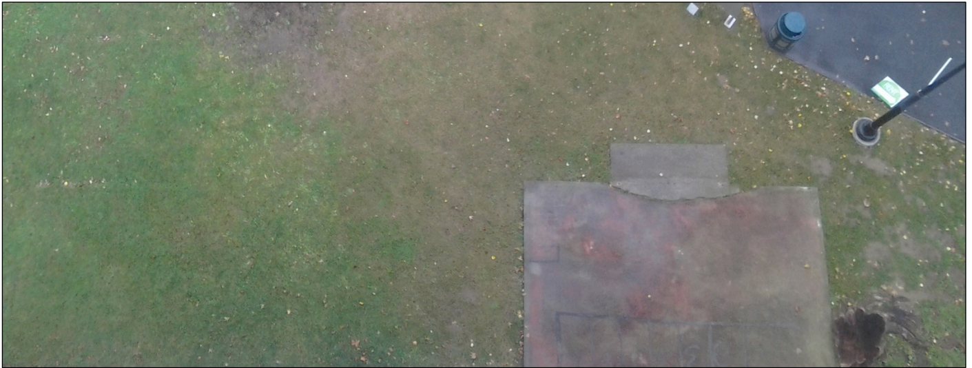
An overhead view of the existing concrete slab on the east side of Whitehead Hall. Our group will make a duplicate of this slab on the left side of the image so we can place two rain storage tanks down instead of one.
