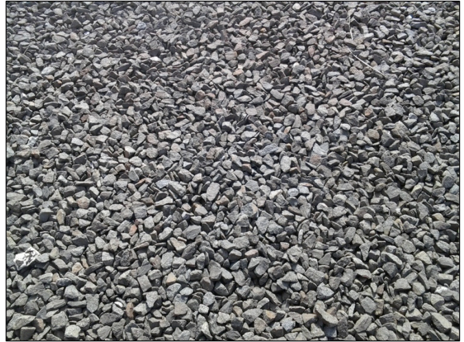
The rock layer on the Whitehead Hall roof.
